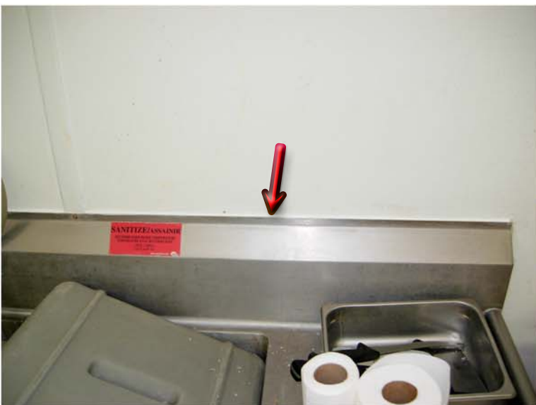
all sinks, walls, coving re-caulked 100% silicon type
