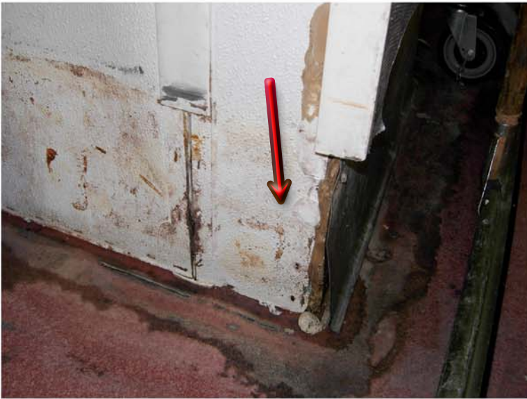
column rotted out needs re-build
