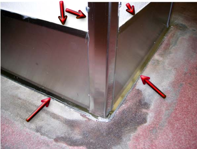
re-caulked with 100% pure silicon caulking
