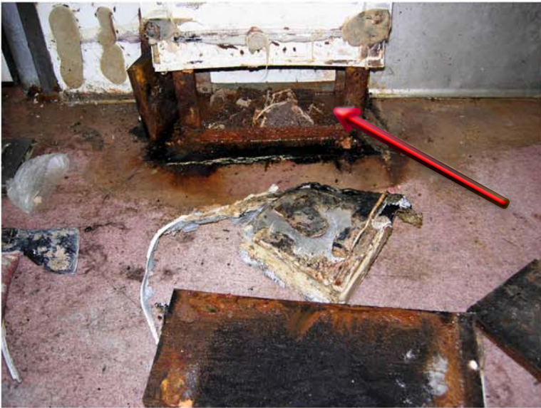
column rotted out needs re-build
