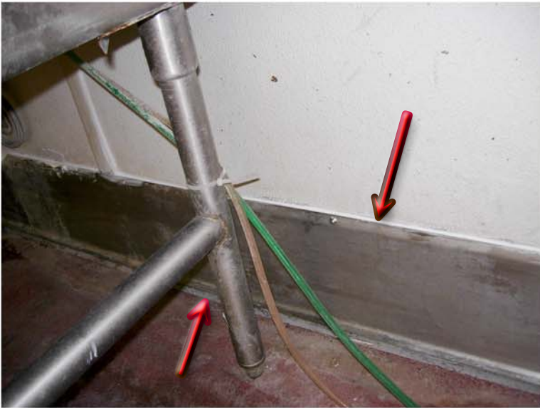
removed all caulking wrong type used
