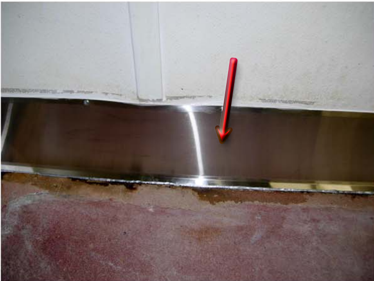
all sinks, walls, coving re-caulked 100% silicon type
