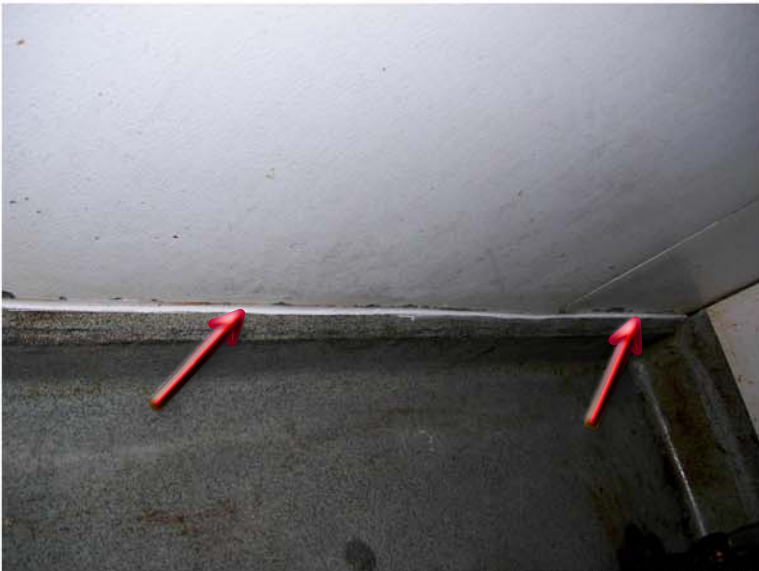
re-caulked with 100% pure silicon caulking
